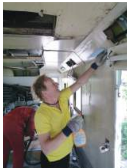
Washing down the interior
