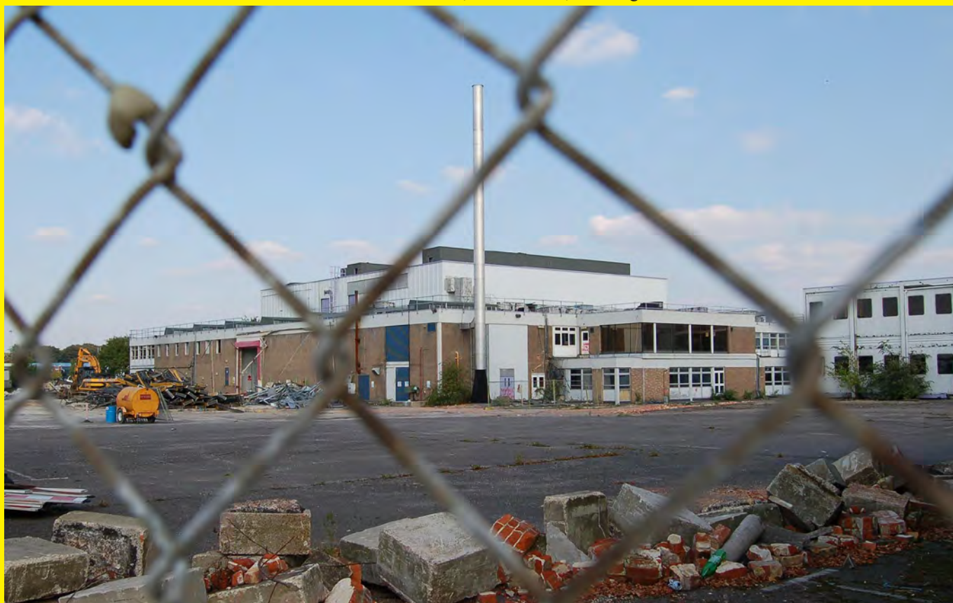
The site of the Northam studios, now derelict, awaiting demolition
