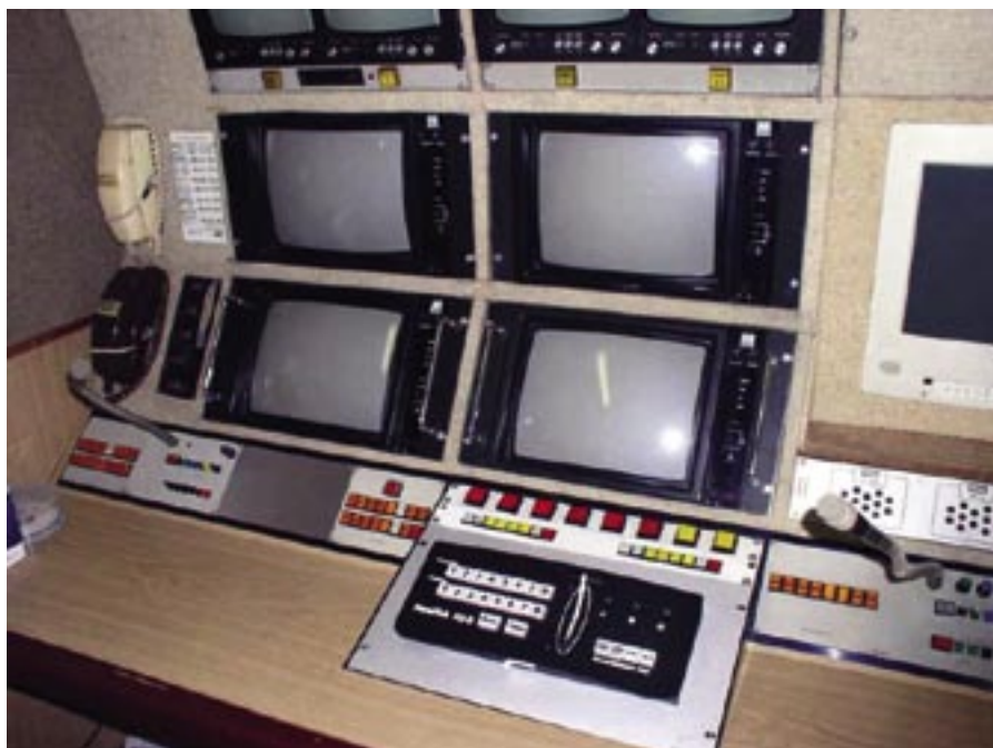
The production area
