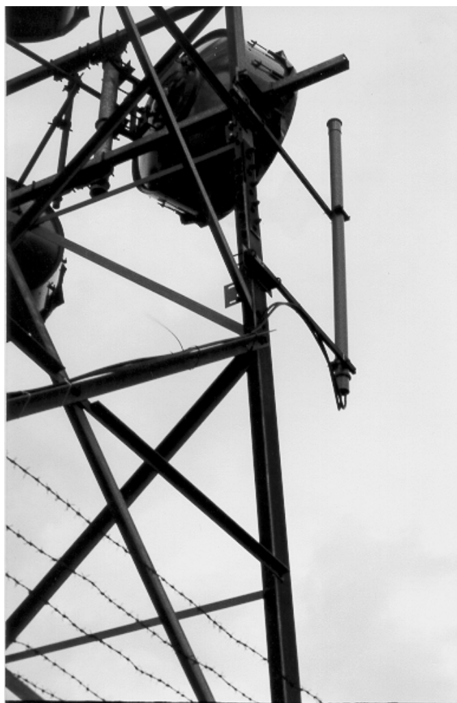
Fig 17. 24cms Dual Alford Slot (in tube) at GB3TM (1994)
