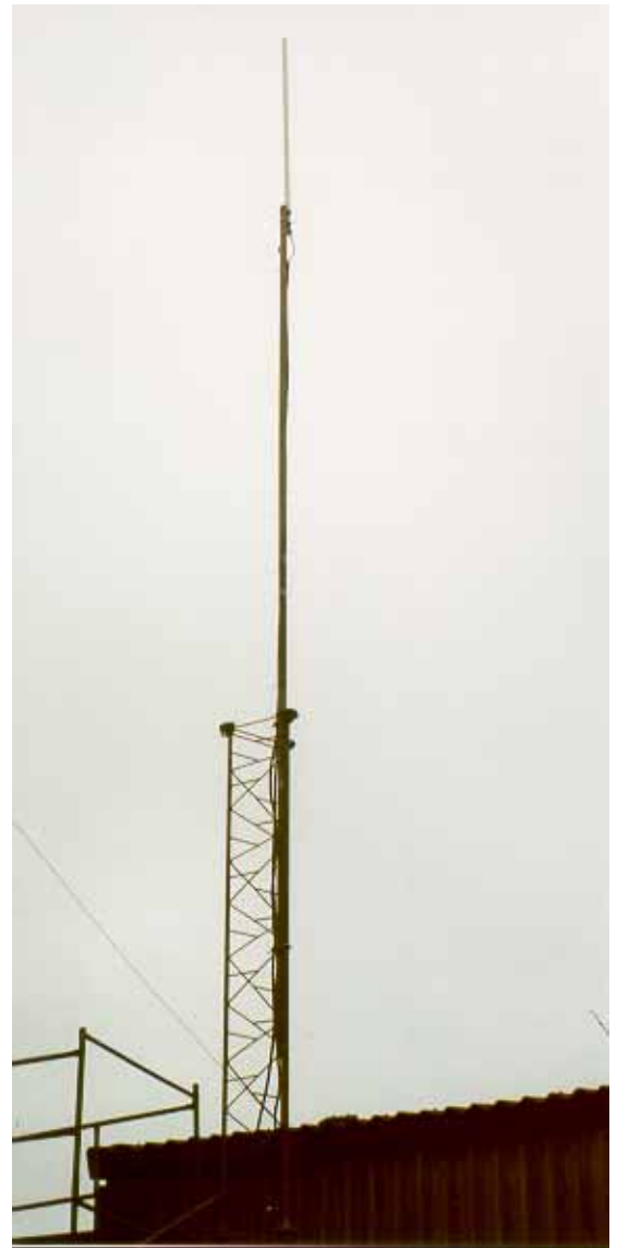
Two views of the dual Alford slot antenna used by the Beacons repeater groups' 1.3GHz ATV repeater. See 'TV on the Air' for more details.
