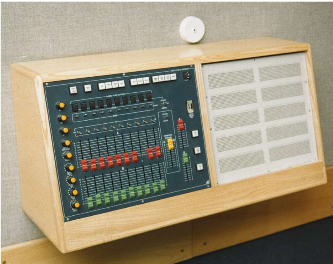
Electrician's set-up control panel and pin patch for checking out installed lanterns during the rigging time.
